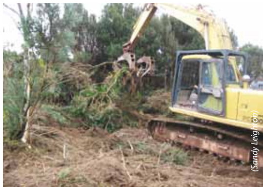
Root raking gorse with an excavator, Zeehan, Tasmania
